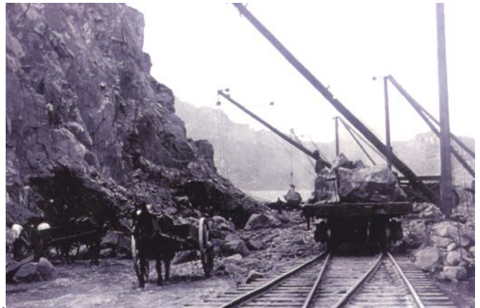
Loading rock at the quarry, notice the rock tongs at center lifting a rock onto a flatbed car.
